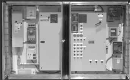
Pad Mounted Control Packages
