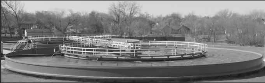
Wastewater Treatment Solutions
